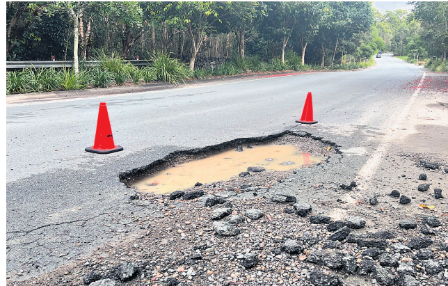
File image of a pothole along Peregian Springs Drive from the February weather event. Photo: Contributed
