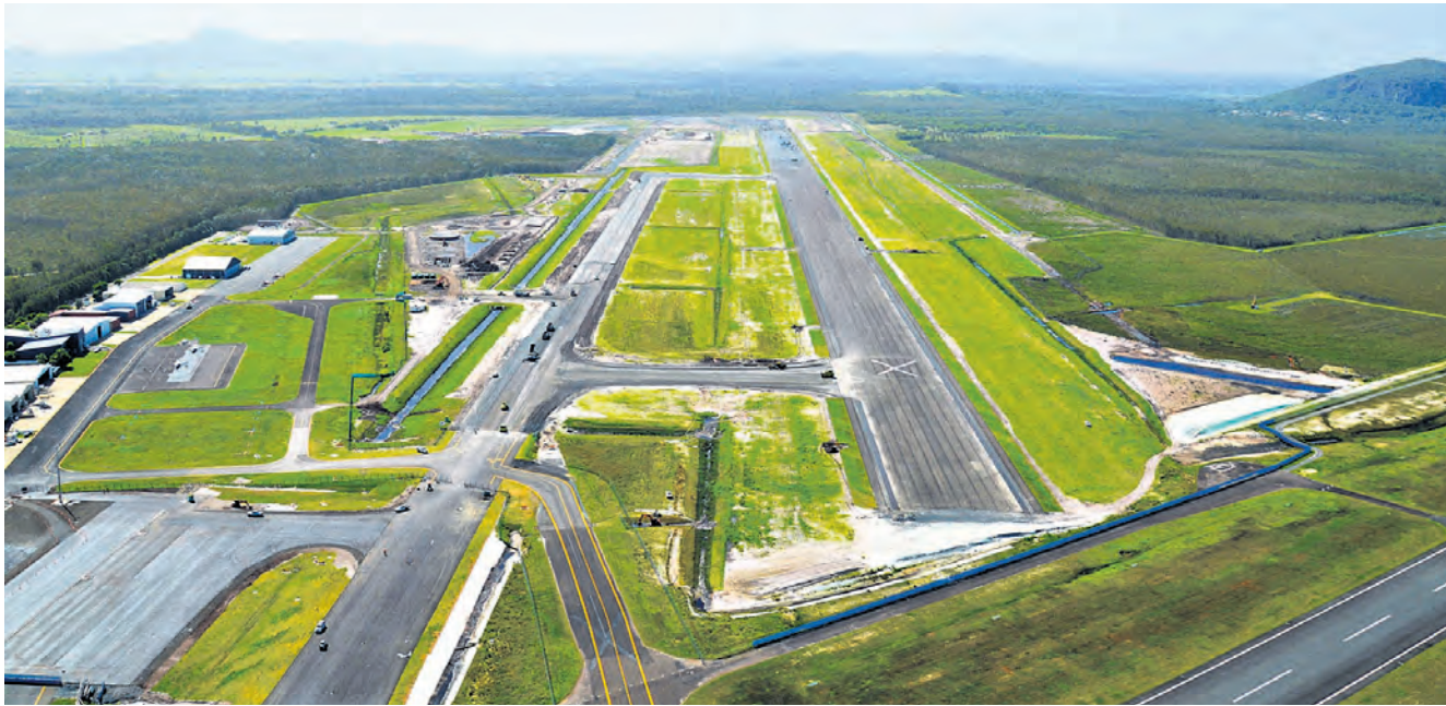
An aerial view of the new Sunshine Coast Airport runway, which was scheduled to be completed by May 21. Heavy rain over late summer and the fallout from the pandemic will now see the runway officially completed on June 14. Photo: Contributed
