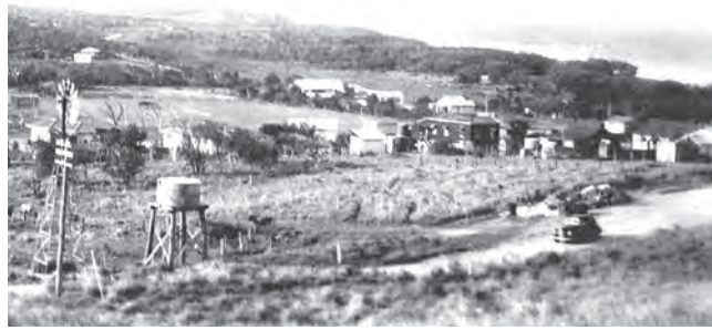
Historical records and anecdotes show that periods of severe dry and a lack of rainfall have been a constant over the past century in our region - this tank in Beach Road supplied water to the campground from the 1940s as a result of a lack of rainfall. Photo: Windolf collection.
